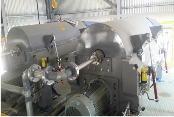
Effluent water application
