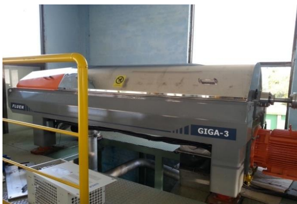
Sewage water application
