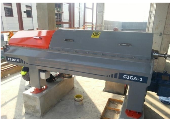
Bio water application
